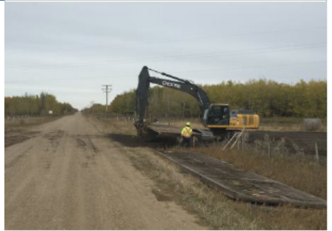
Excavator replacing rig mats – SF 38 – Oct 4, 2018
