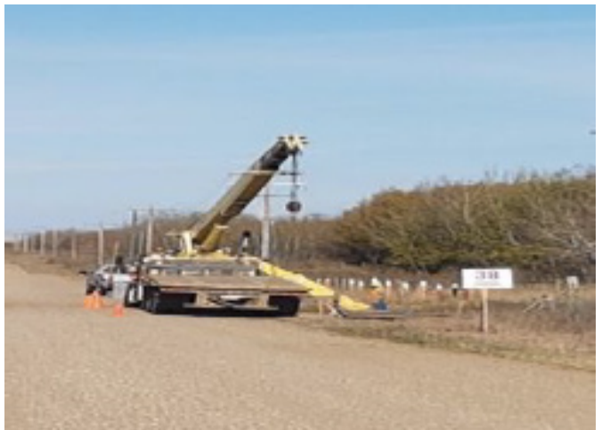
Lowboy with crane loading mats – SF 38 – Oct 6, 2018
