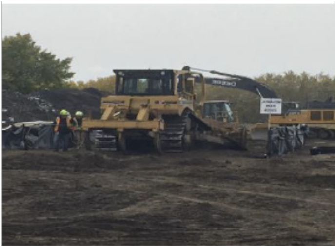
Utility crew cleaning station – SF 37 – Oct 2, 2018
