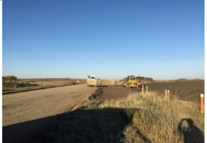
Mechanic starting dozer crew in safety meeting – SF 61 – Oct 6, 2018
