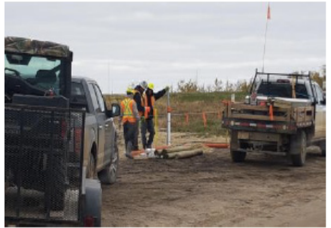
Fencing Crew – SF 7 -Sept 30, 2018
