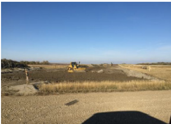
Dozer shaping subsoil - SF 62 -Oct 5, 2018
