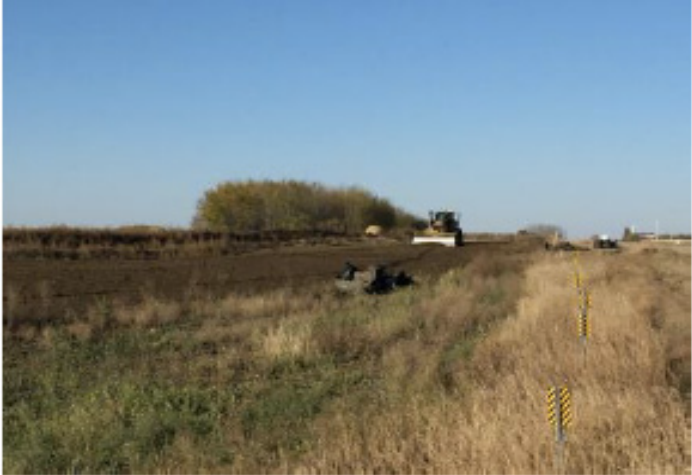
Dozer shaping subsoil - SF 54 - Oct 6, 2018
