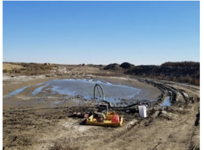
Crews water pumping – SF 44 – Oct 6, 2018
