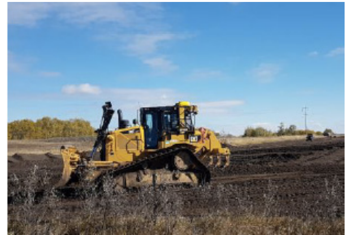
Dozer decompacting subsoil – SF 38 – Oct 3, 2018
