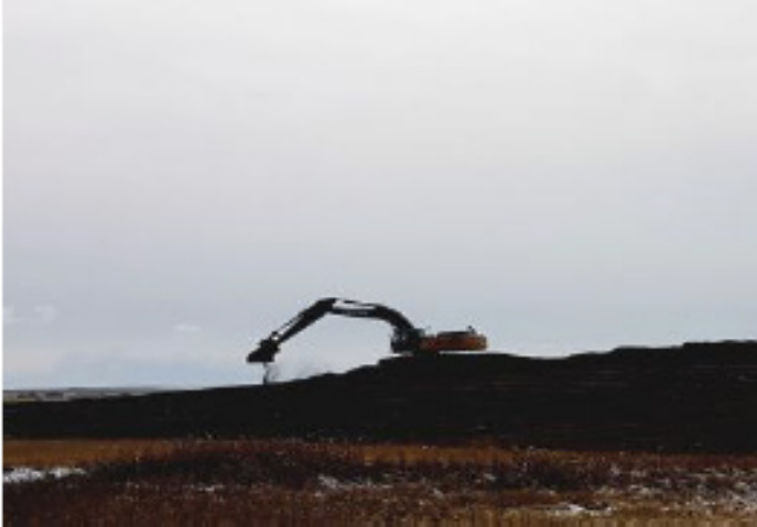
Excavator moving topsoil back onto ROW – SF 36 – Oct 2, 2018
