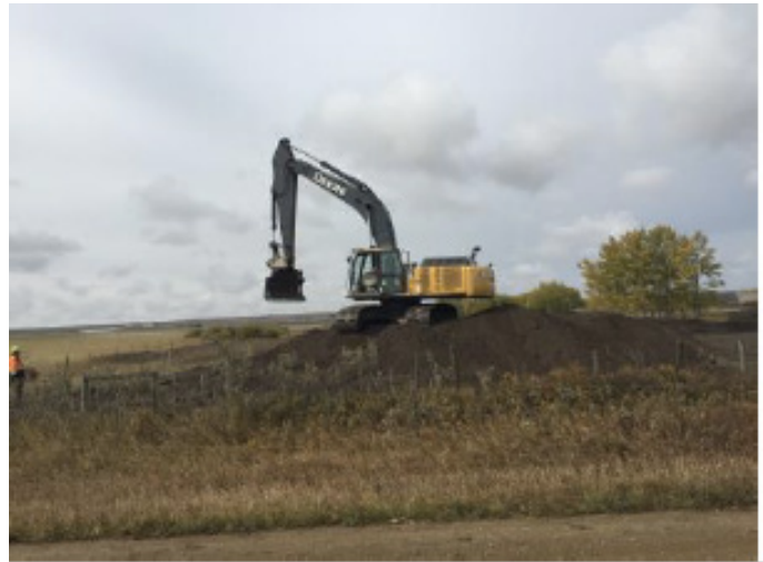
Excavator taking down topsoil – SF 36 – Oct 2, 2018
