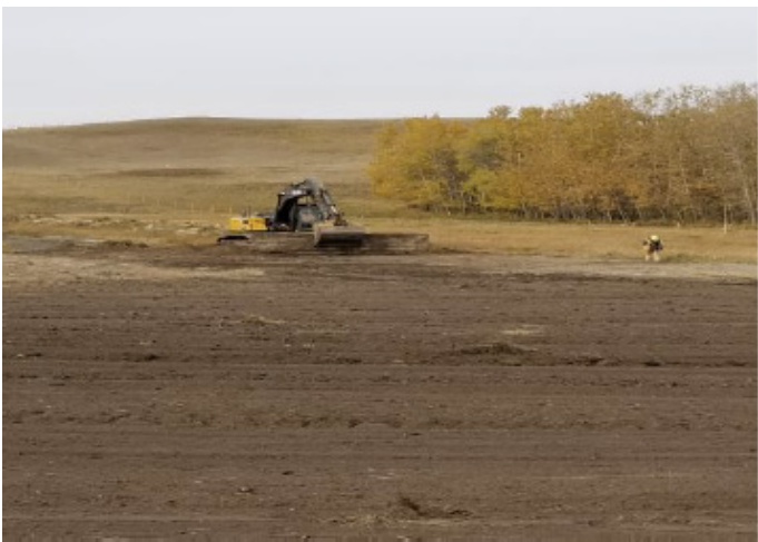
Excavator leveling topsoil with rig mats - SF 29 -Oct 4, 2018
