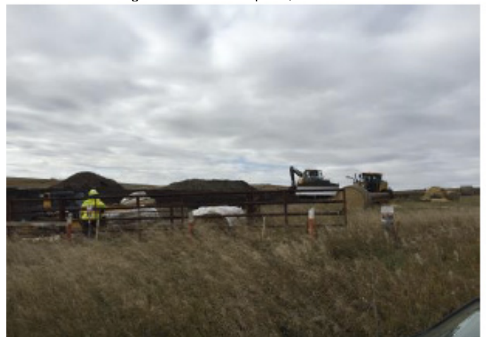
Topsoil and utility crew – SF 36 - Sept 30, 2018
