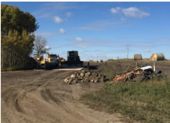
Rock debris at cleaning station - SF 38 -Oct 3, 2018
