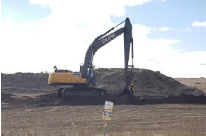
Excavator working topsoil with flat blade – SF 36 - Sept 30, 2018
