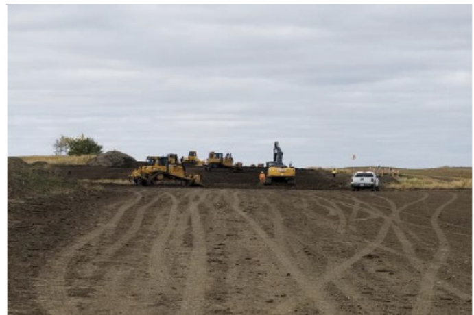
Excavator hotline ramp removal – SF 27 – Sept 30, 2018
