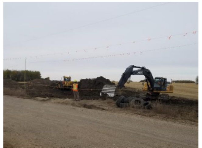
Excavator access ramp removal – SF 54 – Oct 4, 2018
