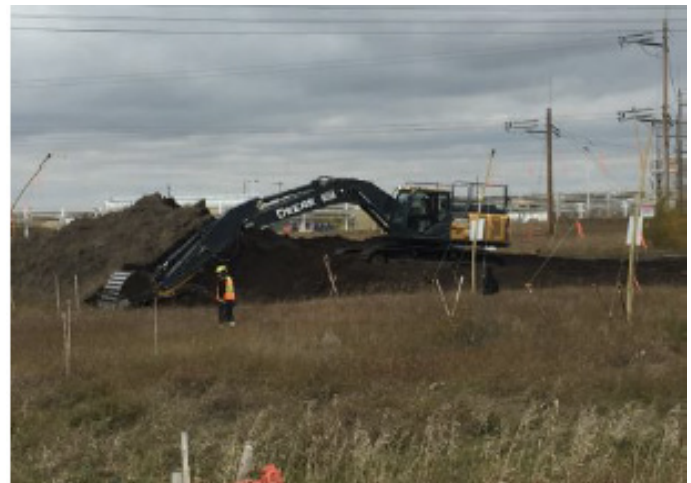
Excavator taking down topsoil – km 54+700 – Oct 1, 2018
