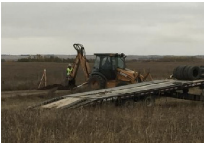
Texas gate replacement – SF 62 – Oct 1, 2018
