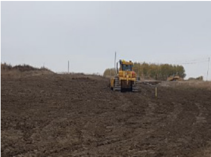
Dozer working subsoil - SF 54 -Oct 4, 2018
