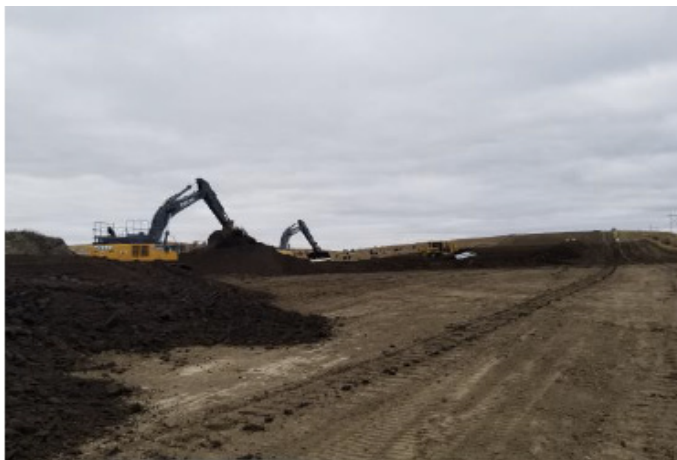
Dozer and excavator on ROW – SF 36 – Sept 30, 2018
