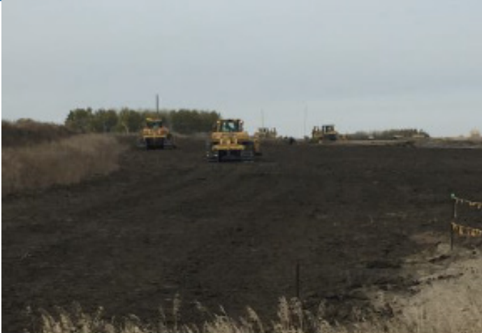
Dozer shaping sub soil - SF 53 -Oct 4, 2018
